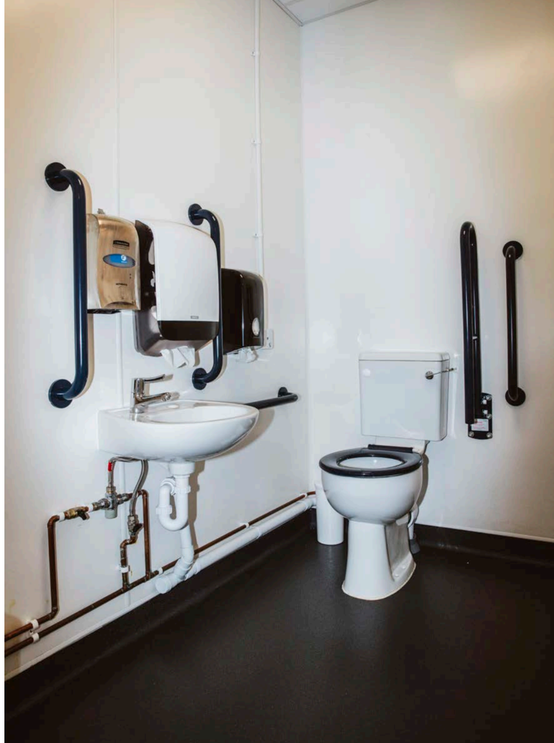
Photo: Accessible Toilet
