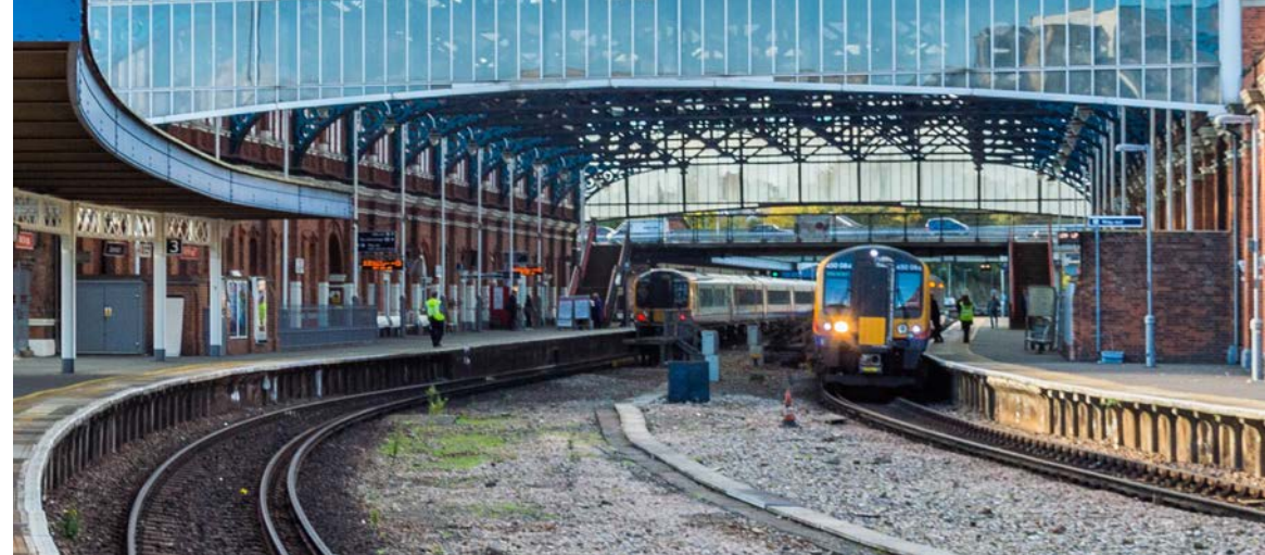
Photo: Bournemouth Station
